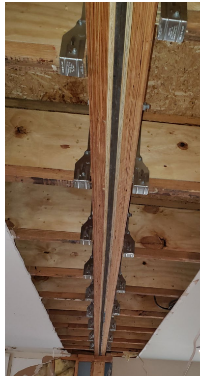
Beam in ceiling replaces 18' of load-bearing wall.
